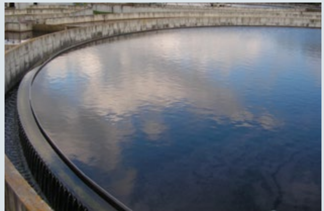
3 pic. Secondary sludge settling tank before and during the use of GREASOLUX
